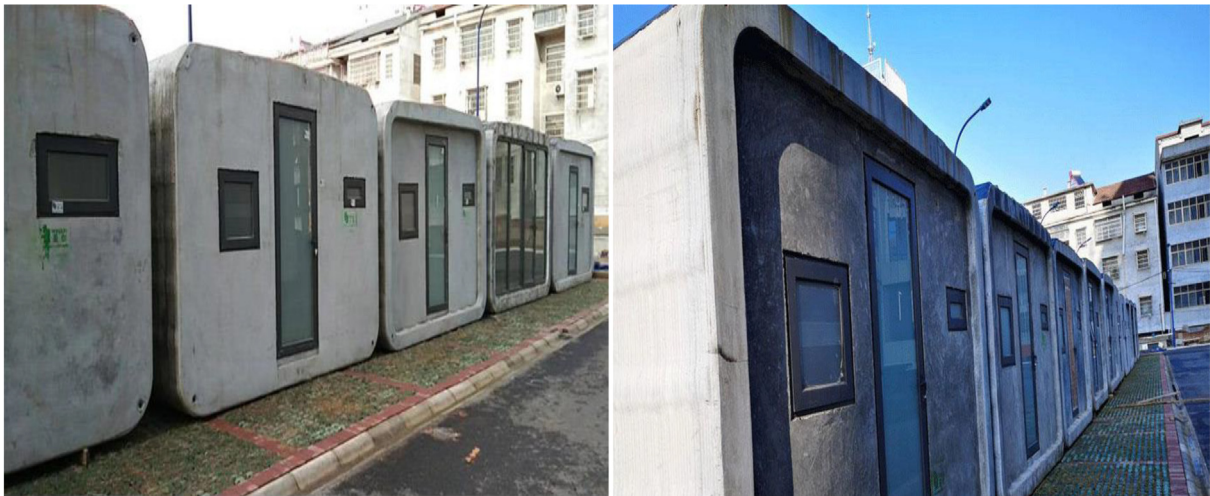
Fig. 3. Houses developed for isolation in Xianning, China.
